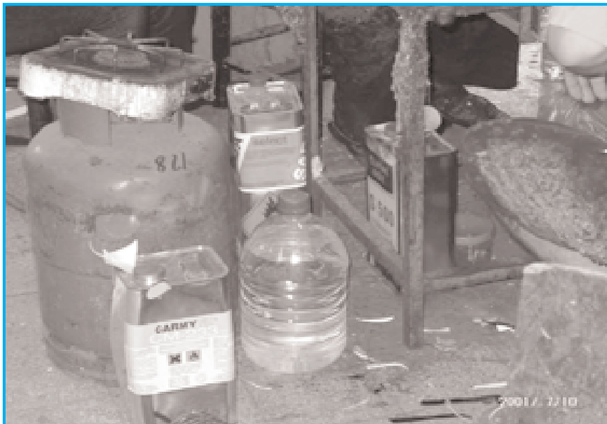
Photo 16: Chemicals are haphazardly stored. This is a potential risk to workers health in their working environment (see the source of gas, ignition and flammable liquids stored side by side). This is by no means acceptable for both health and safety purposes.
