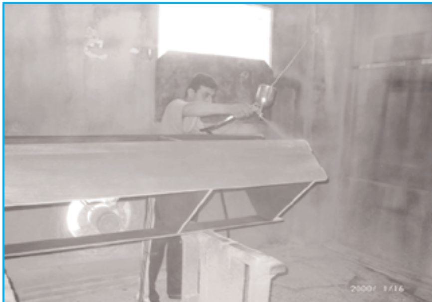
Photo 8: The total absence of local exhaust ventilation and the utilisation of general ventilation is an unacceptable practice. It does not protect the worker. In some instances in fact if badly designed may increase worker exposure to chemicals (see general ventilation in the middle of photo).
