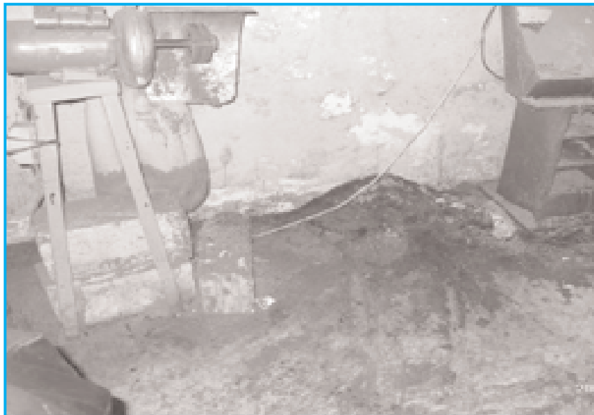
Photo 4: General hygiene in industrial premises are not acceptable. This may increase overall potential exposure to occupational hazards.
