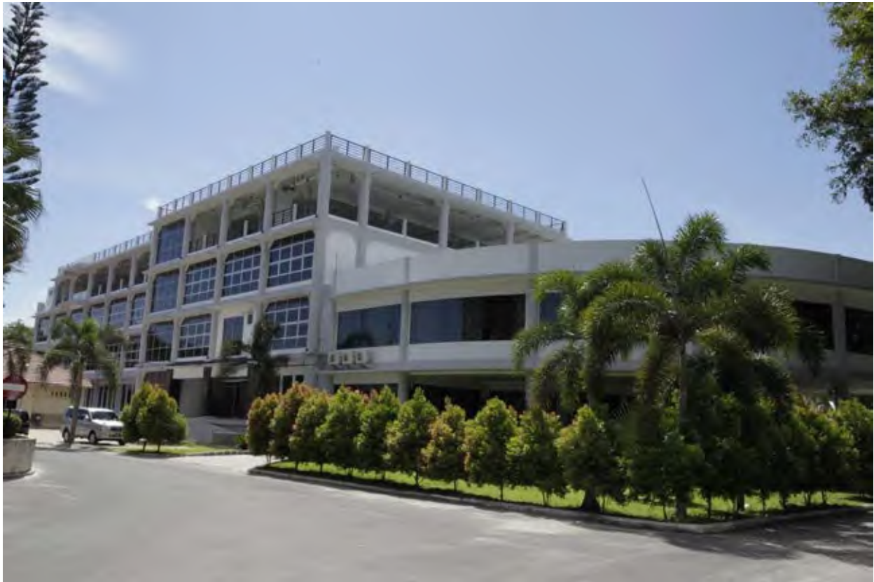
Shelter at the Governor's Office, Padang
