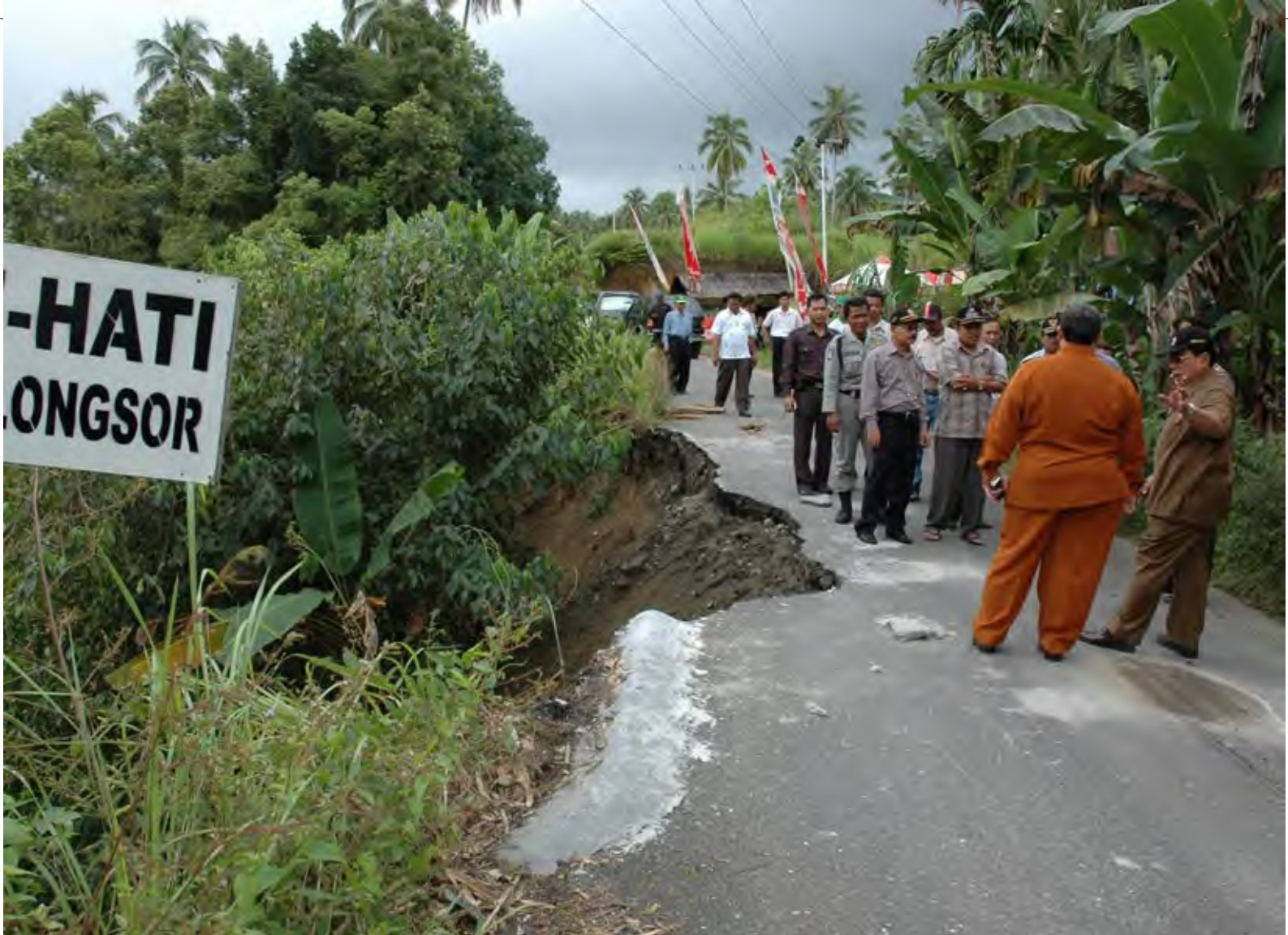
Landslide in Padang Pariaman. Source : BNPB
