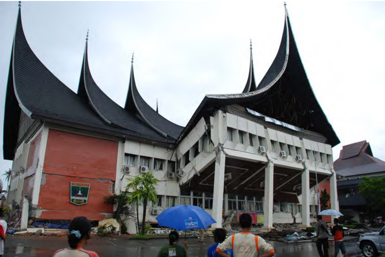
West Sumatra parliament office was severely damaged by earthquake in Padang City. Source : BNPB
